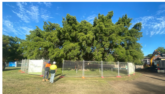
Fencing set up to protect the TPZ around this tree from ongoing development.
