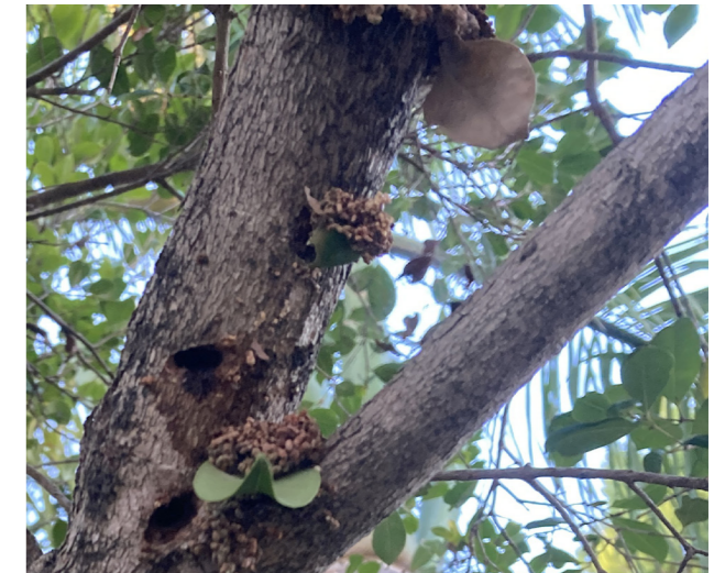
Example of what a wood borer infestation looks like from the outside.
