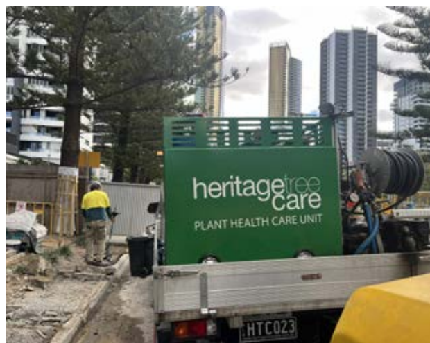
Plant Health Care unit deployed to a live construction site, supporting retained council trees with construction impacts through the construction phase.
