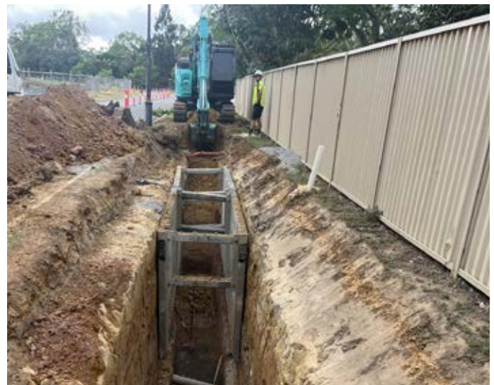
Deep service trench through a road reserve, with private tree impacts assessed and managed ahead of excavation.
