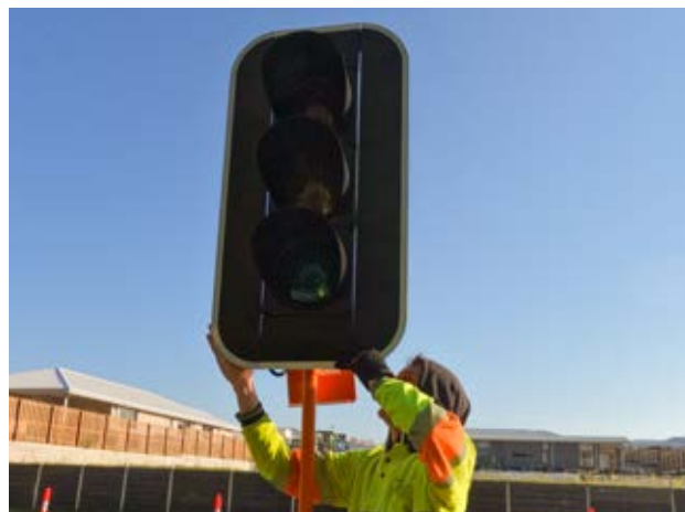
In some instances traffic lights may need to be set-up to ensure the safe and efficient flow of traffic at all times of the day.
