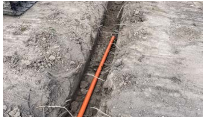
Trenching for electrical conduits monitored by a Project Arborist within a Tree Protection Zone, with alignment set to avoid structural roots.
