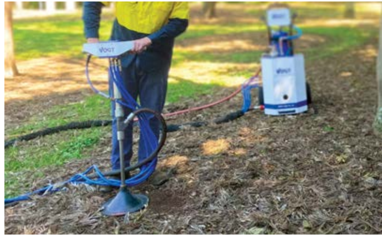
VOGT needle that is injected into the ground and is used to disperse the air and other material into the soil.
