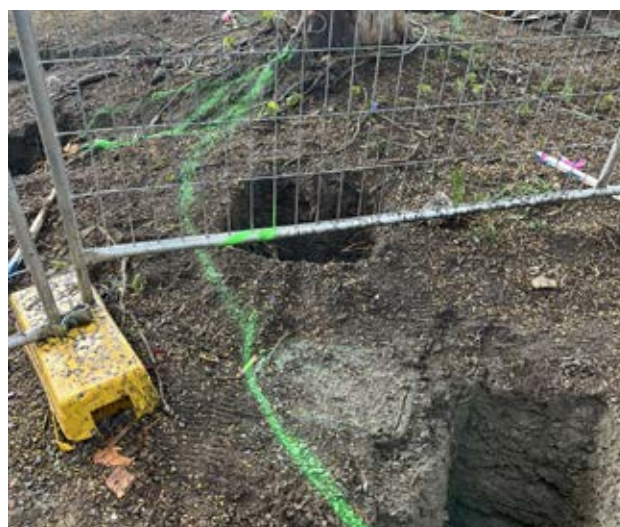
Marked roots within the Tree Protection Zone of a retained tree for pier and beam seating ahead of excavation, guiding works away from structural roots.
