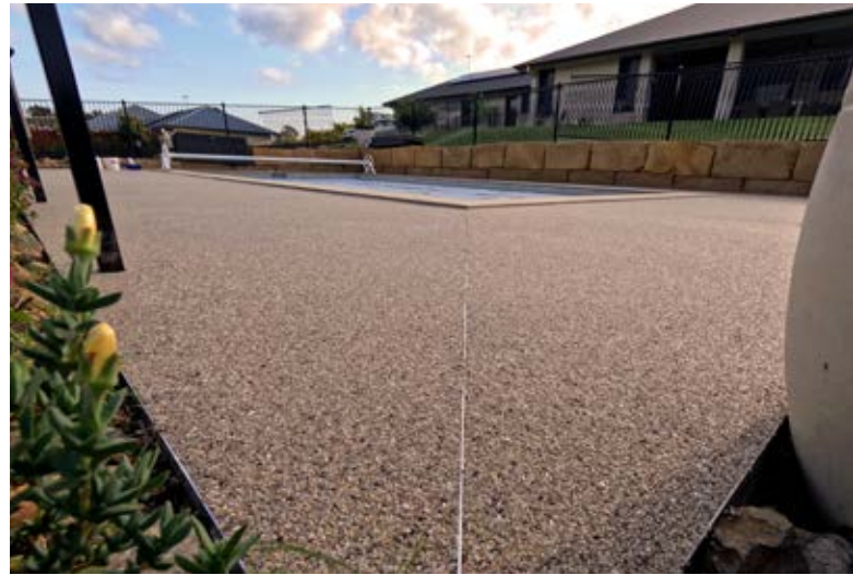
Pool surround with Porous Paving installed. This material allows liquids to freely flow through it, providing a fantastic solution to prevent puddles from forming.
