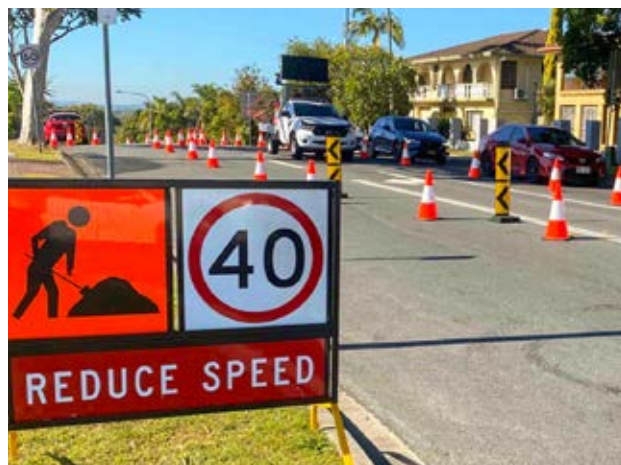
Long-term signage helps maintain safety and assist the flow of traffic even when traffic controllers are not present on site, ie when works are expected to take over a day to complete.
