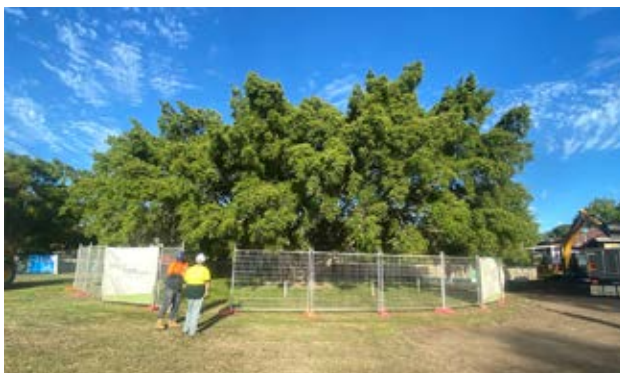
Fencing set up to protect the TPZ around this tree from ongoing development.
