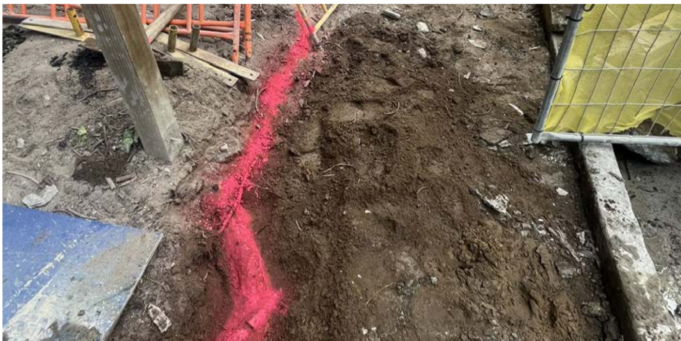
Non-destructive excavation and service marking within a Tree Protection Zone, allowing paving infrastructure to be installed without compromising tree stability.
